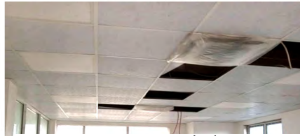
VRF System at FIRS Egbeda Lagos
