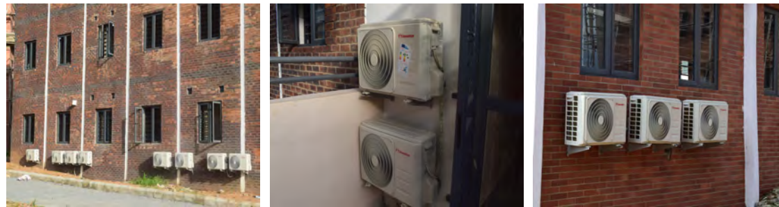
Supply & Installation of units at Alethea University, Ago-Iwoye
