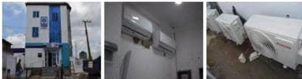
Supply & Installation of units at All Branches of Lotus Bank
