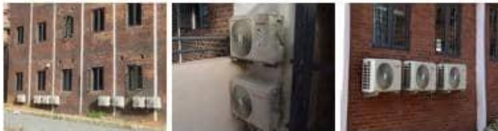
Supply & Installation of units at Alethea University, Ago-Iwoye
